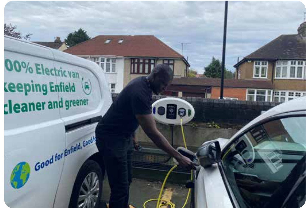
Electric vehicle charging point
